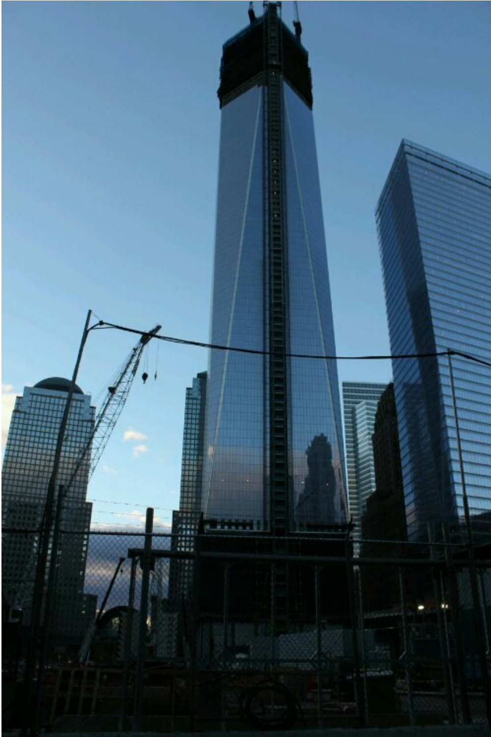
Rebuild well underway
