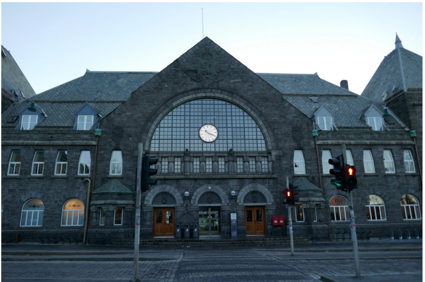
Bergen Railway Station
